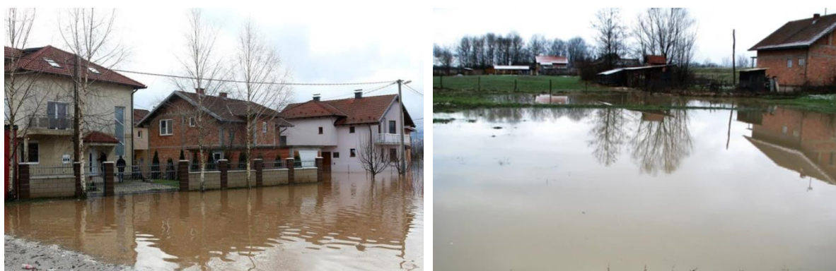
Figure 27: Flooded buildings and Krusevac-Djunis road in 2016 60
