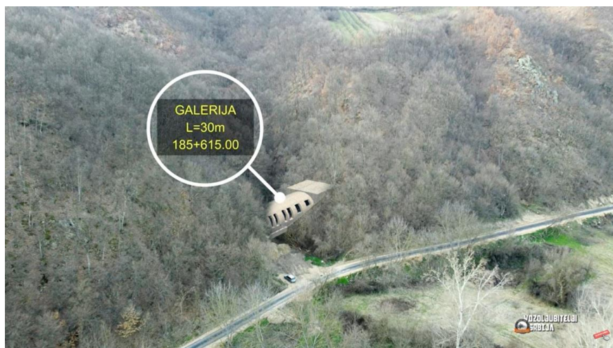
Figure 41: Gallery between the entrance portal of Tunnel no. 4 and entrance portal of Tunnel no. 5
