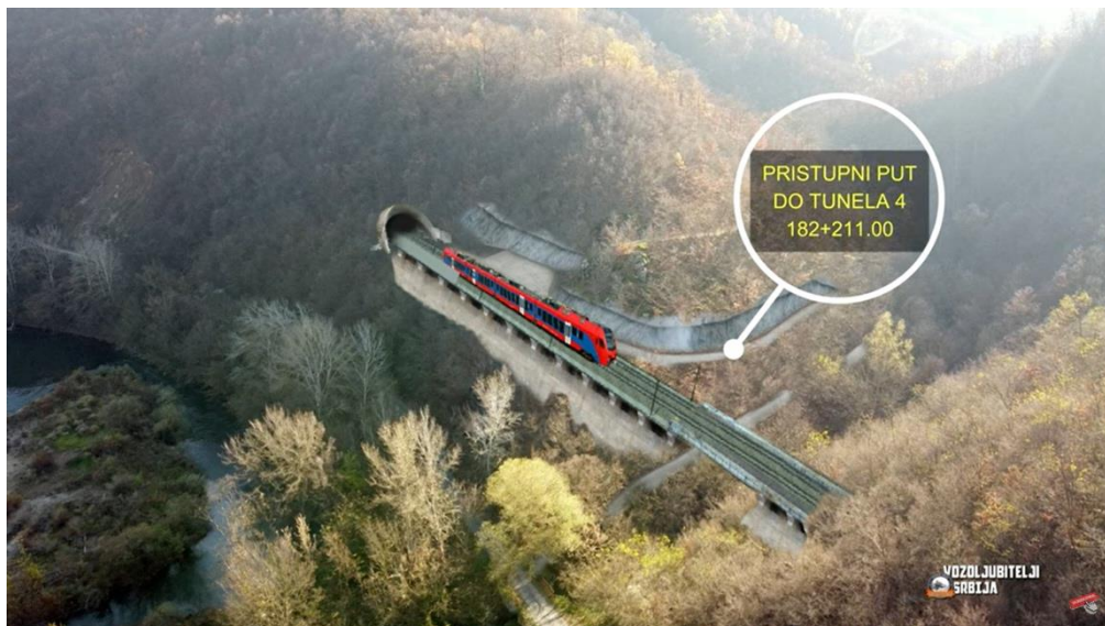
Figure 40: Entrance portal of Tunnel no. 4 with access road
