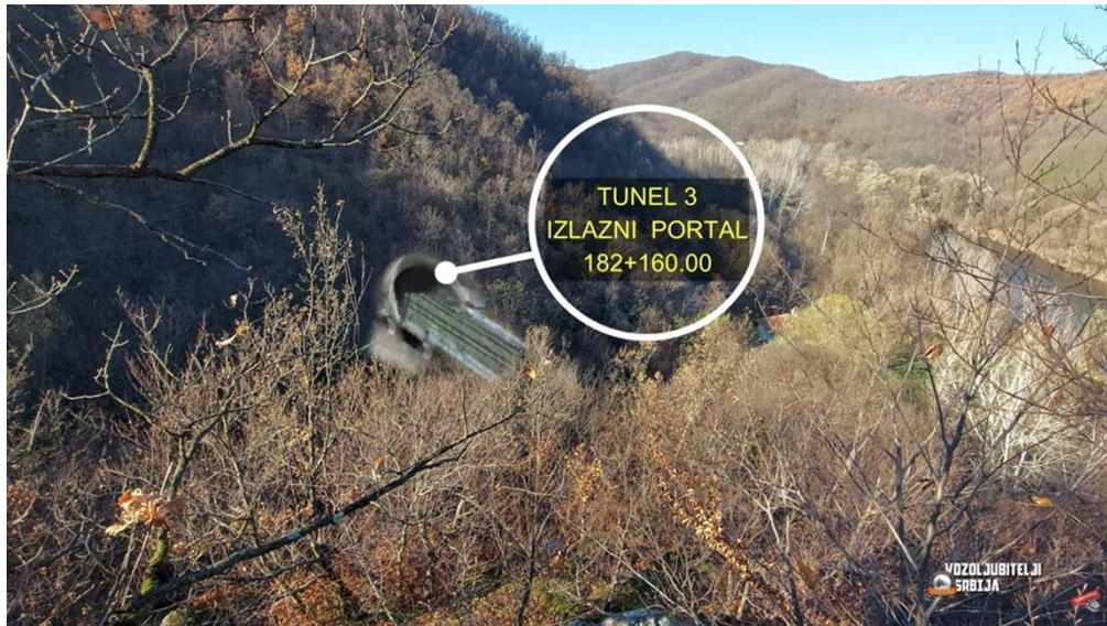
Figure 39: Exit portal of Tunnel no. 3
