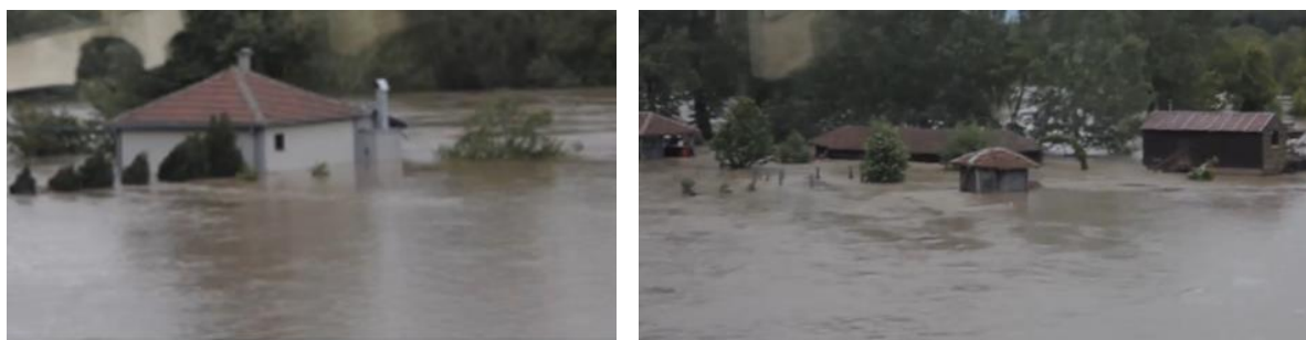
Figure 26: Flooded buildings and agricultural areas along the Stalac-Krusevac road in 2014 58
