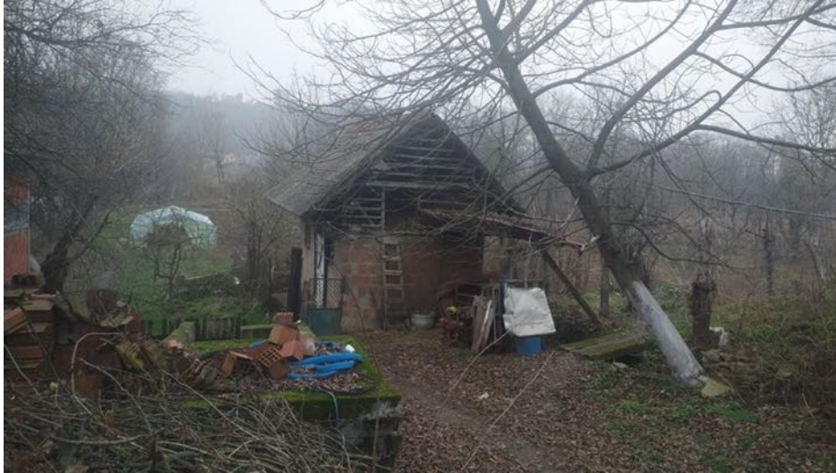
Non residential structure
