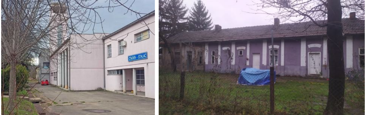
Five SRI owned apartments, within the Stalać Railway Station complex
