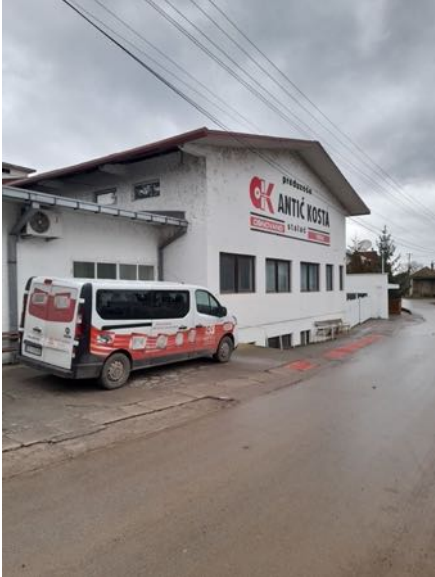
Metal processing factory, outside and inside
