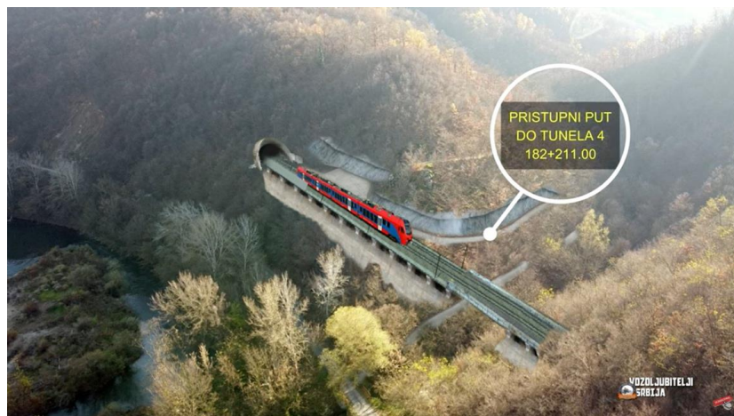
Figure 6: Entrance portal of Tunnel no. 4 with access road
