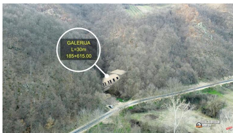
Figure 7: Gallery between the entrance portal of Tunnel no. 4 and entrance portal of Tunnel no. 5
