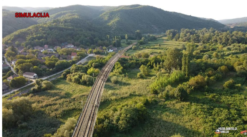
Figure 4: Crossing of the existing railway with the new one in the settlement of Djunis
