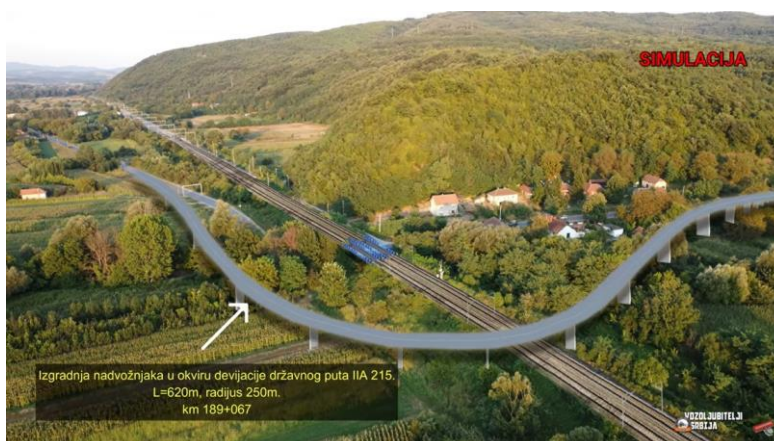
Figure 2: Route of the future railway alignment with the construction of an overpass within the realignment of the state road in the Djunis settlement
