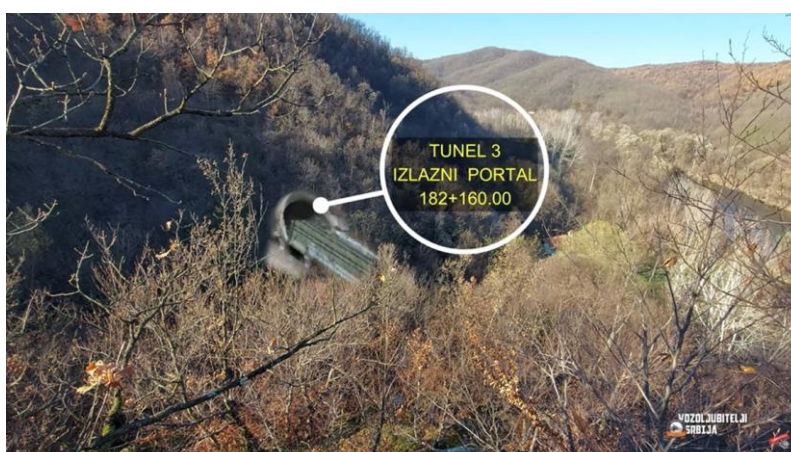
Figure 5: Exit portal of Tunnel no. 3
