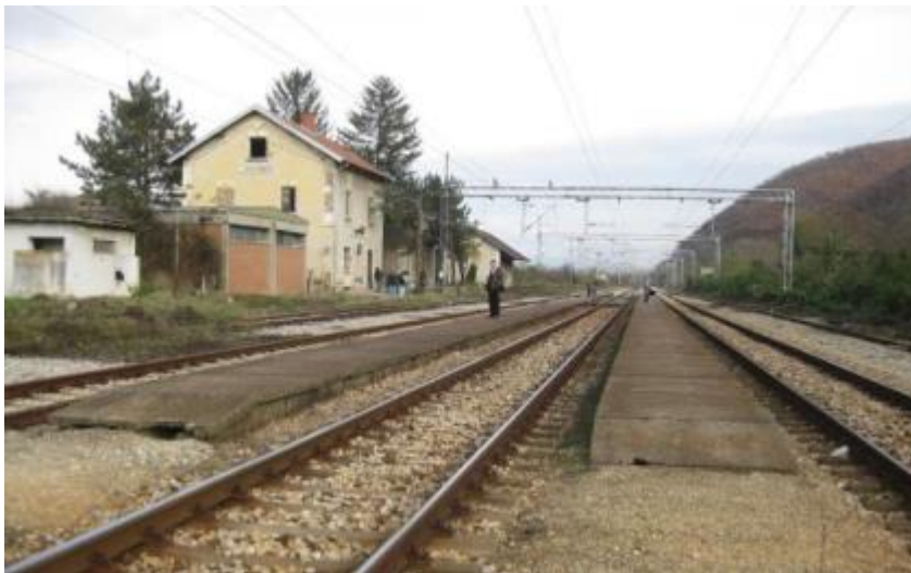
Figure 3 Đunis station – present state
