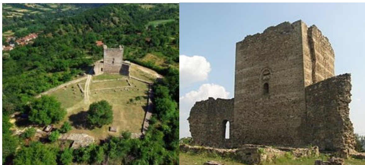
Figure 31 Town Stalać (L) and Tower Todor of Stalać (R)
