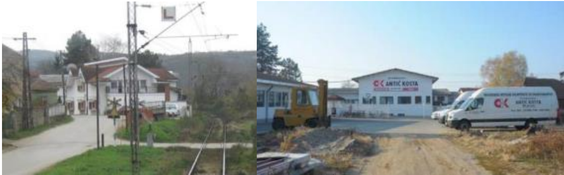
Figure 35 Properties situated within the right-of-way of the new route
