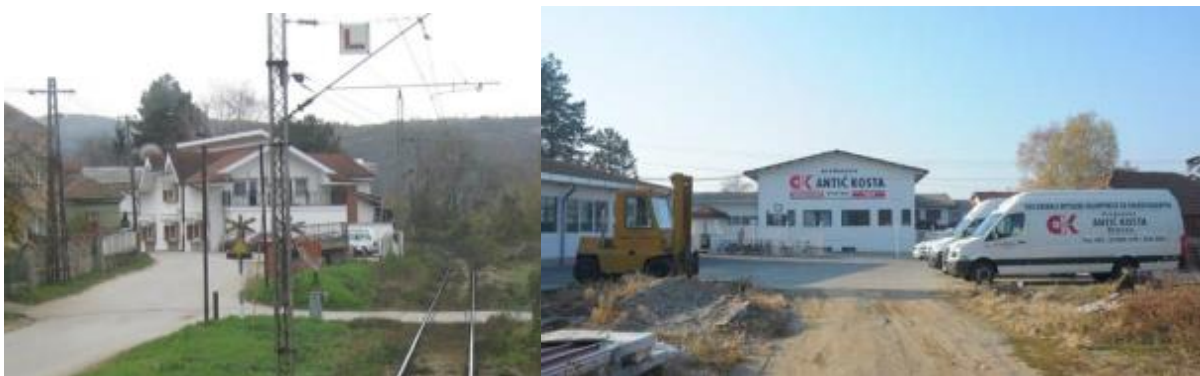
Figure 3 Properties situated within the right-of-way of the new route
