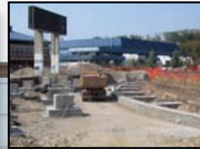
3 CAIR STADIUM RECONSTRUCTION SECOND PHASE
