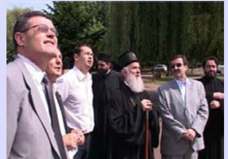
Patriarch Irinej and Niš City officials visiting ongoing works on the Church "Emperor Constantine and Empress Helen"
