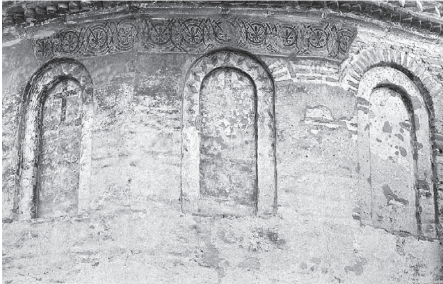
Fig. 4 A detail of a façade of the Patriarchate of Peč with painted decorative ornaments (author)
