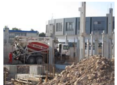
Construction of New Stadium
