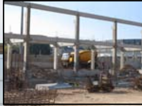
2 ČAIR STADIUM RECONSTRUCTION
