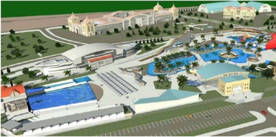
Lozni Kalem Location Design After Completed Construction
