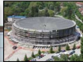
4 ARENA ČAIR RECONSTRUCTION PROGRESSING ACCORDING TO...
