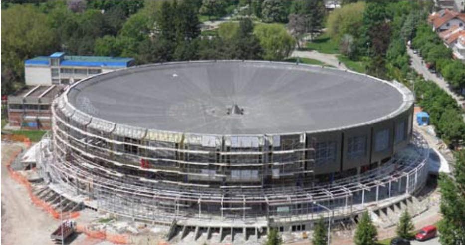
Arena Čair Reconstruction progressing according to planned dynamics
